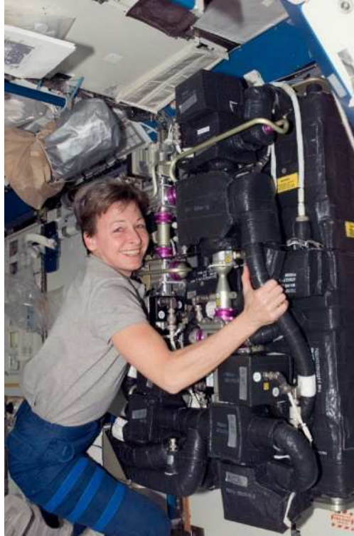
Figure 8: Astronaut Peggy Whitson on ISS Expedition 16 Performing In-flight Maintenance on the Carbon Dioxide Removal Assembly
